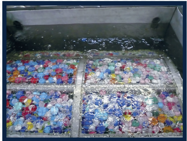
Fig. 2 - The reaction cell is 100% plunged in the sewage. Denitrifying bacteria grow as biofilm on the carriers promoting nitrates reduction to nitrogen gas.
